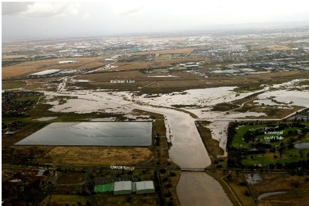
Melway Ref: 53-K-12 (looking north)
