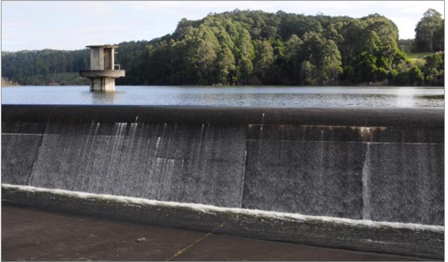
Figure 3. West Barwon Reservoir spillway.
