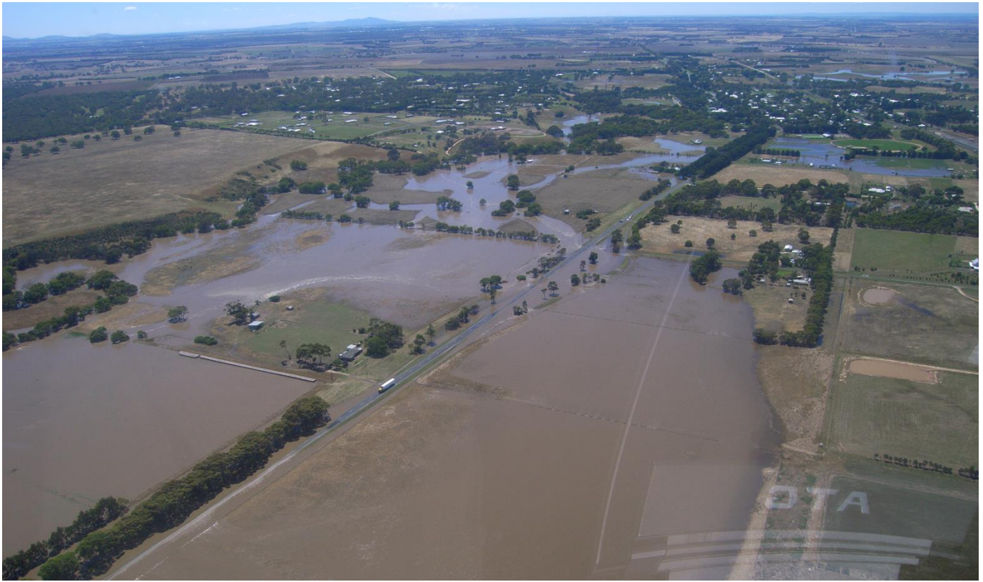
Figure 13. Flooding impacting the Hamilton Highway, looking east towards Inverleigh during the 2011 flood event.
