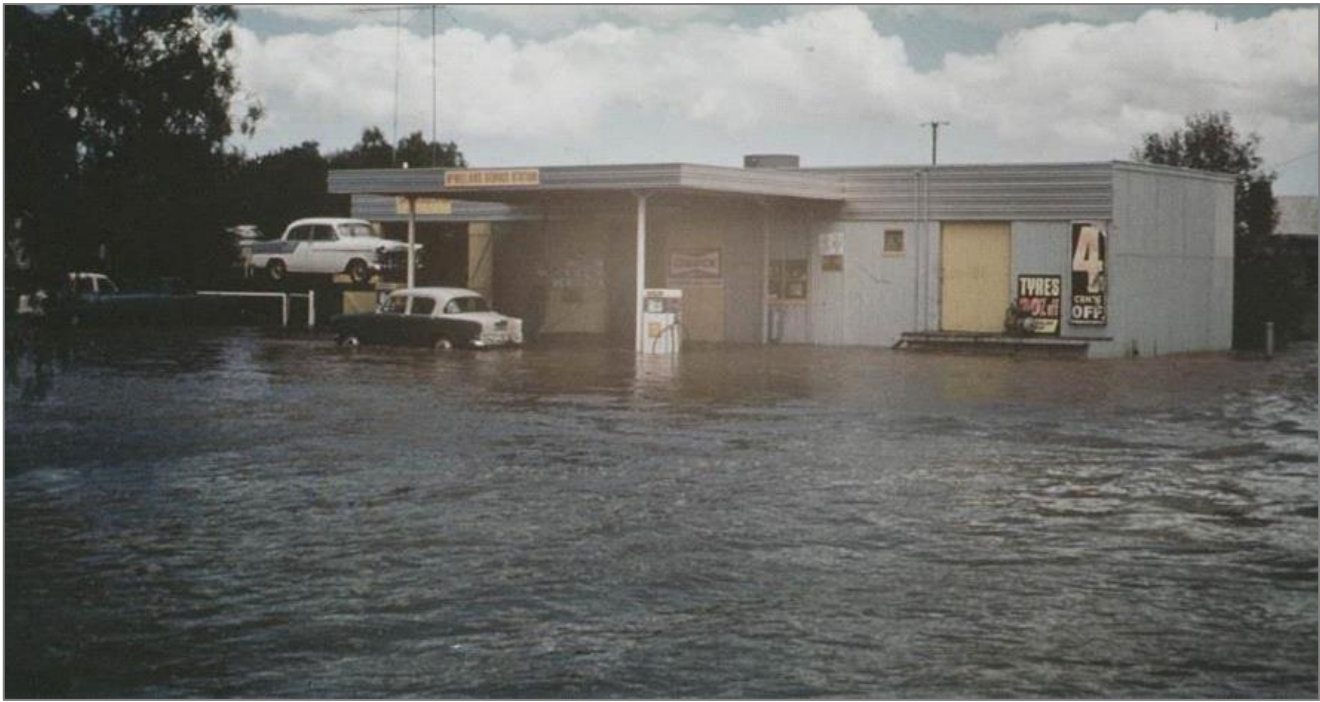
Figure 9. Flooding impacting the Inverleigh Service Station, 19 High Street during the 1973 flood event.
