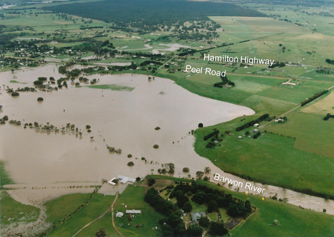
Figure 12. Flooding southeast of Inverleigh during the 1995 flood event.
